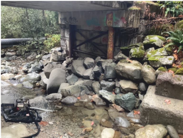
Right Bank Abutment when facing downstream
