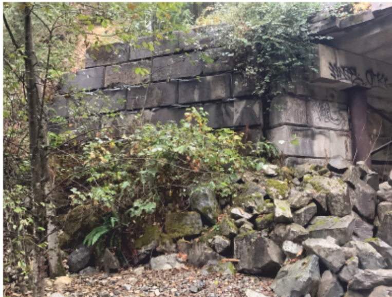
Downstream right wing wall
