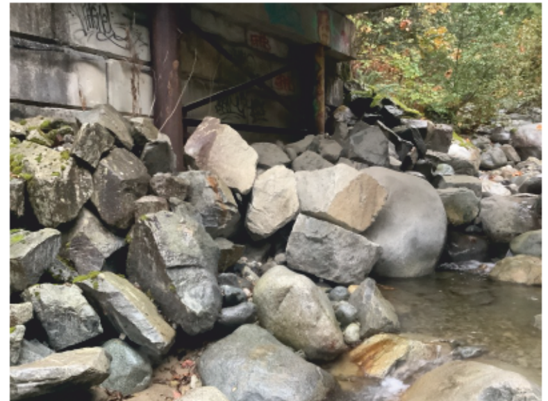
Right Bank Abutment when facing downstream
