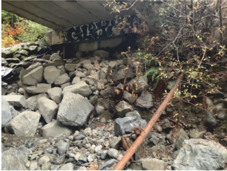
Left Bank Abutment when facing downstream
