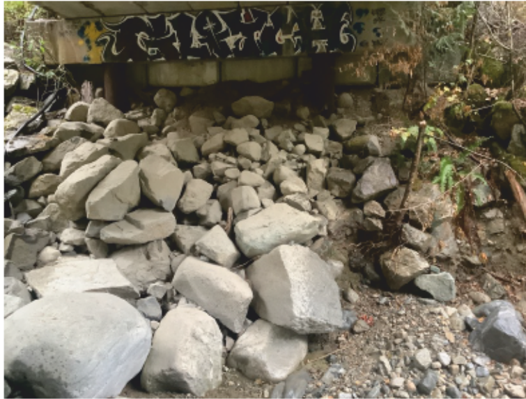
Left Bank Abutment when facing downstream
